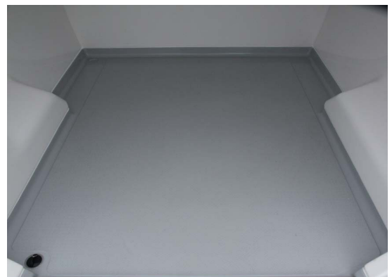
75 mm upturn on floor pan
